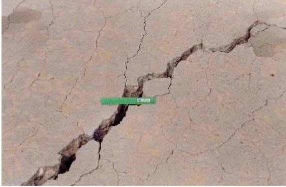
*ASR (alkali-silica reactivity) deterioration of concrete*
