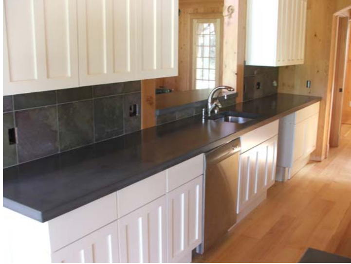
Figure 13 – GFRP Counter Top with Black Pigment and VCASHS
