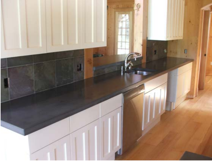
Figure 13 – GFRC Counter Top with Black Pigment and VCASHS
